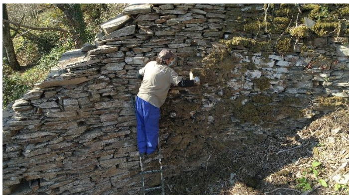
Dry stone masonry work for the restoration of the walls of one of the acquired alvares
